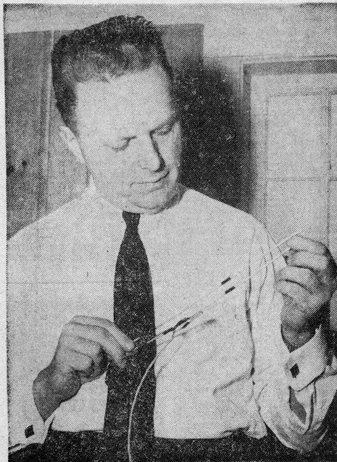
With safer driving as his dream, George Humphrey of Worthington, above, displays his invention the Humphrey E-Z Deicer. The deicer consists of a switch, attached to the dashboard of a car, which when flipped sends an electric current that melts snow and sleet sticking to the windshield wiper.
