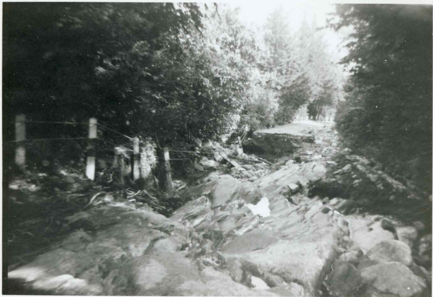
Road in Wottinghamton torn out by flood 1955
