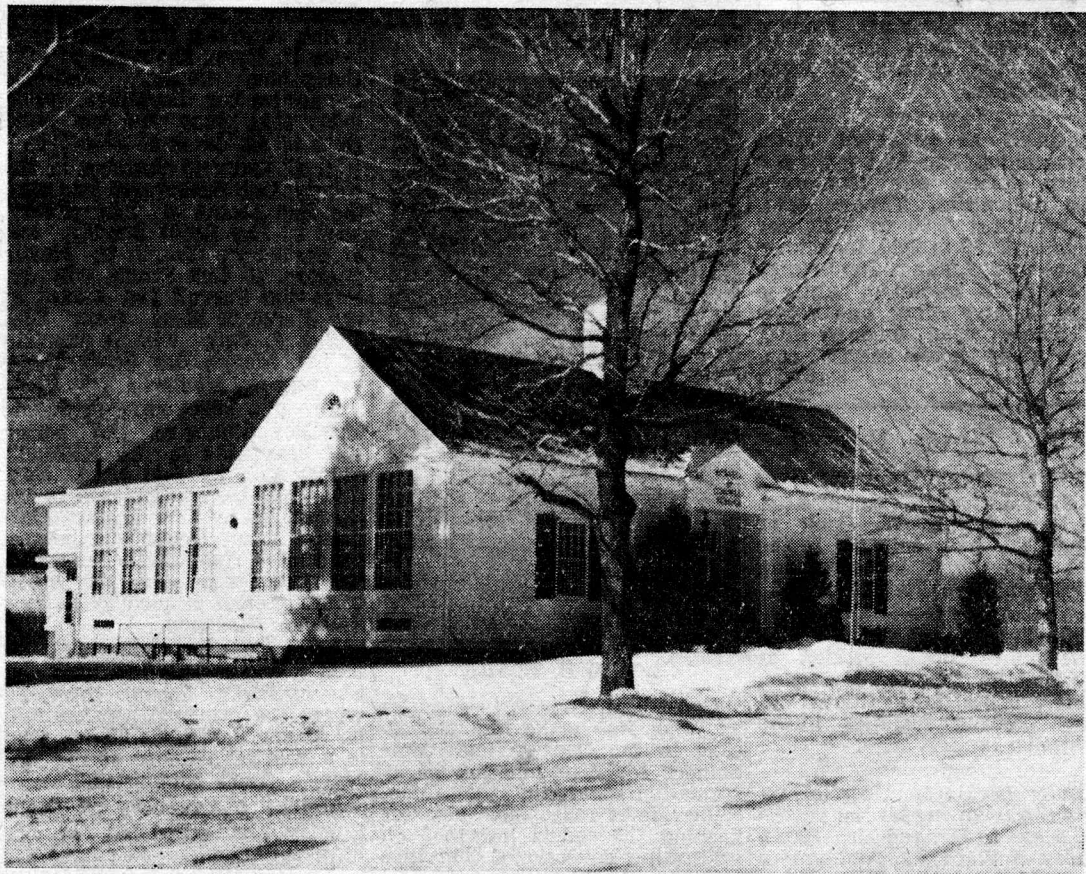
WORTHINGTON—This community's modern Russell H. Conwell School, built in 1941 in the center of town, replaced a two-room makeshift arrangement in the old Lyceum Hall now occupied by the Worthington Health Assn. and two one-room schools similar to the district school pictured below. The well-equipped, fenced playground lacks a brook and trees to climb.
