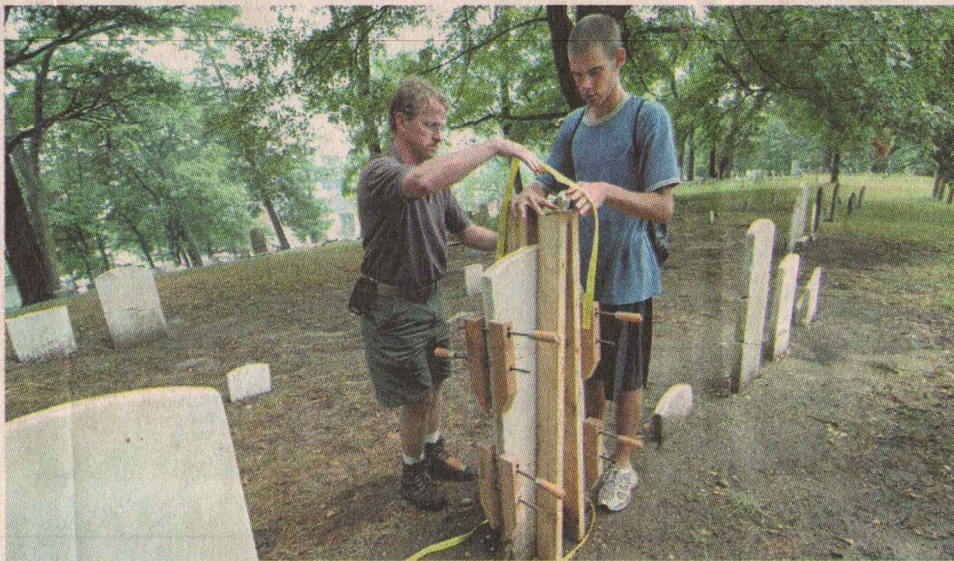
R.I.P. Joel Snodgrass and Morgan C. Davey repaired broken tombstones in Huntington this summer. The cemetery restoration work is expected to continue into next year.
