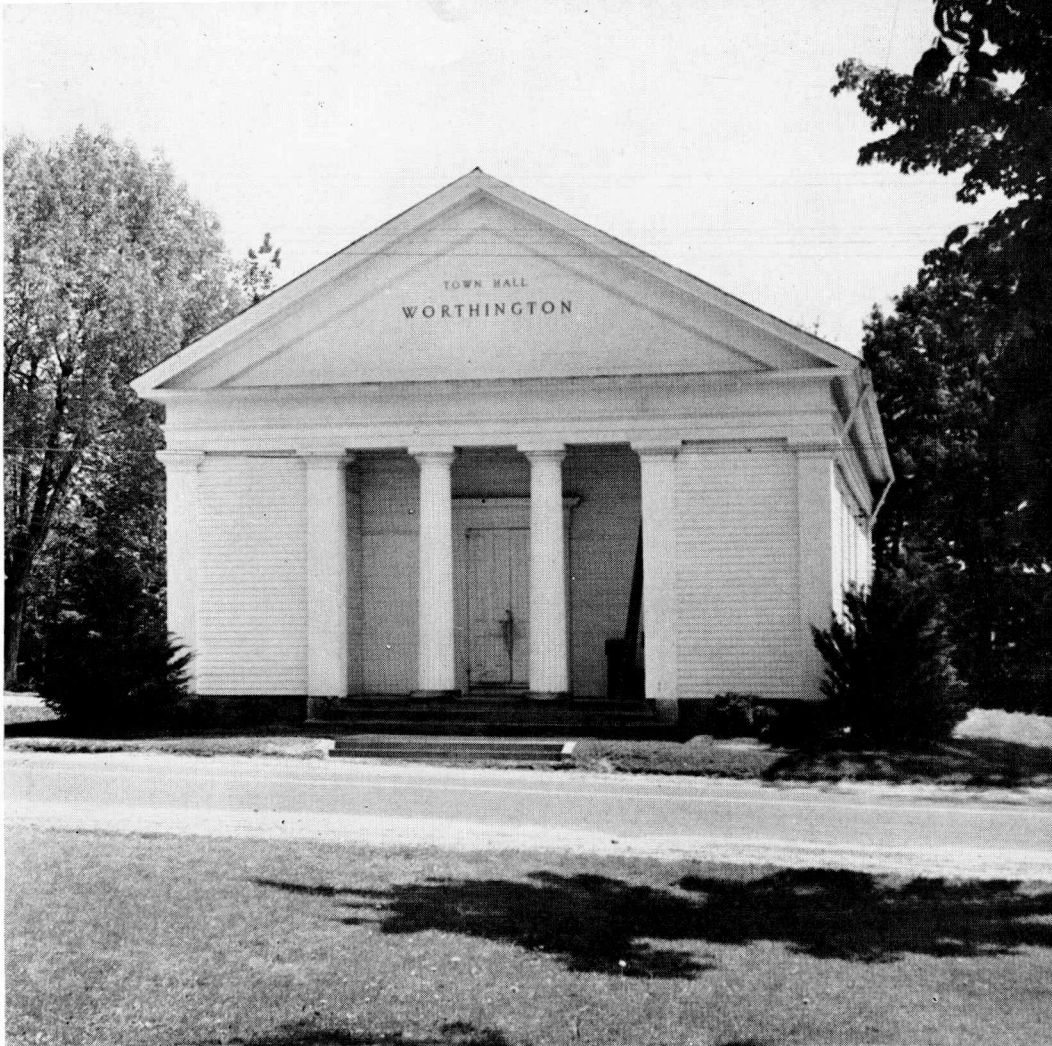
This is the Worthington Town Hall, a typically New England kind of structure with its Grecian columns and white clapboards, a fitting home for Town Meetings. It was here that the first New England Town Meeting—Telephone Style—was held.
