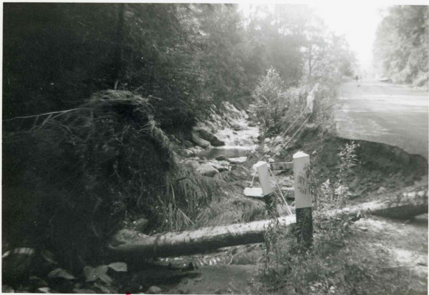
Road to Worthington-Washed out by flood in 1955
