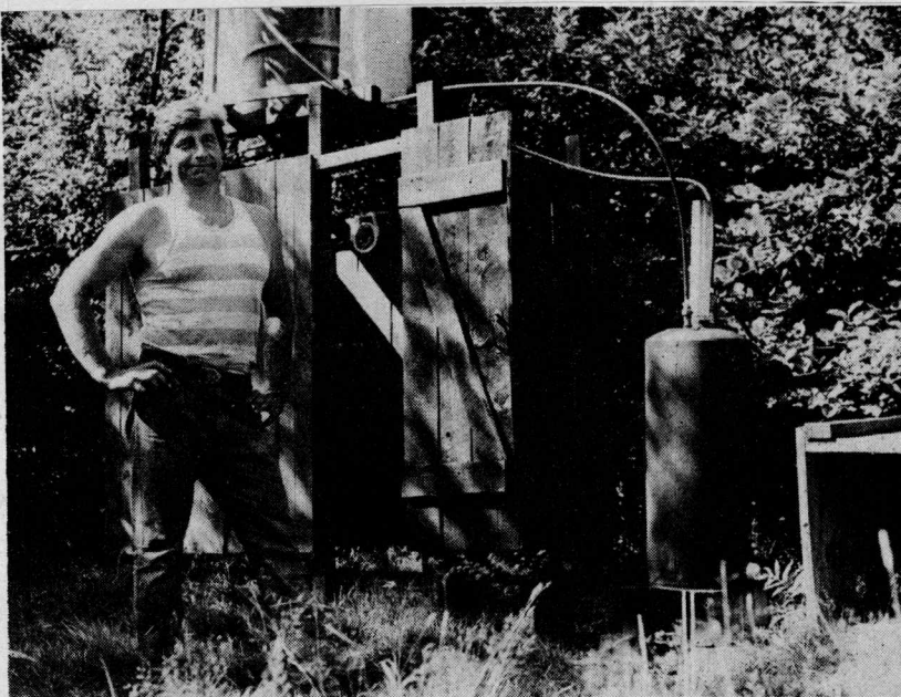
ROBERT COOK shows off the outdoor woodburning hot-water shower, which he assembled from things he found in a junkyard. (Photo by Maureen Fitzgerald)
