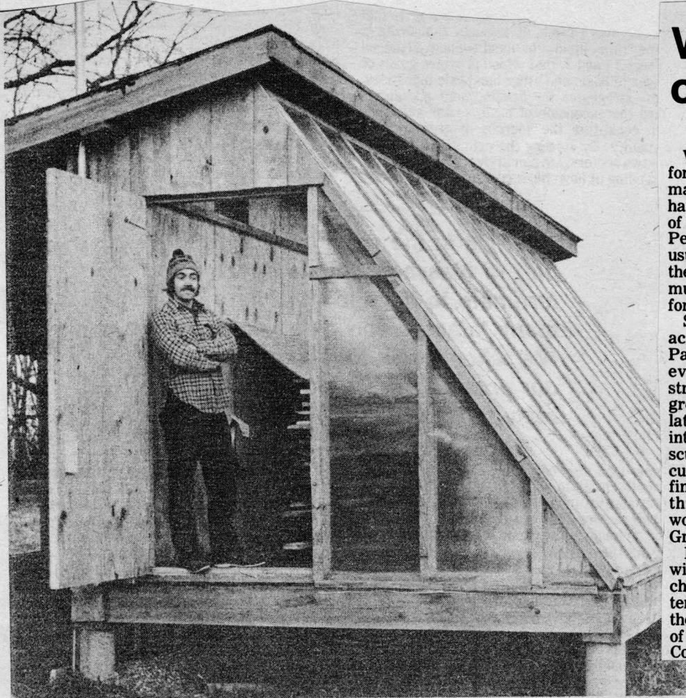
DEANE RYKERSON of Worthington is shown with his solar-powered wood kiln — the only one of its kind in the Northeast. The kiln is used to season hardwood so that it may be used to make finished wood products, like furniture.
